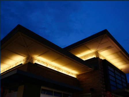
Architectural accent lighting
