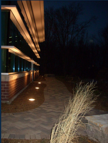
Ground mounted lighting of facade
