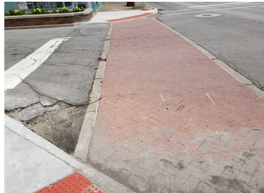
Existing Condition: Stamped asphalt crosswalks have faded, lots of cracking, most in fair condition Opportunity: Replace existing crosswalks with new decorative paving to create consistent pedestrian crossings
