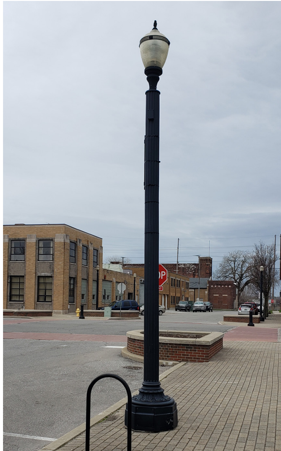
Existing Condition: City standard pedestrian lights Opportunity: Replace with new city standard
