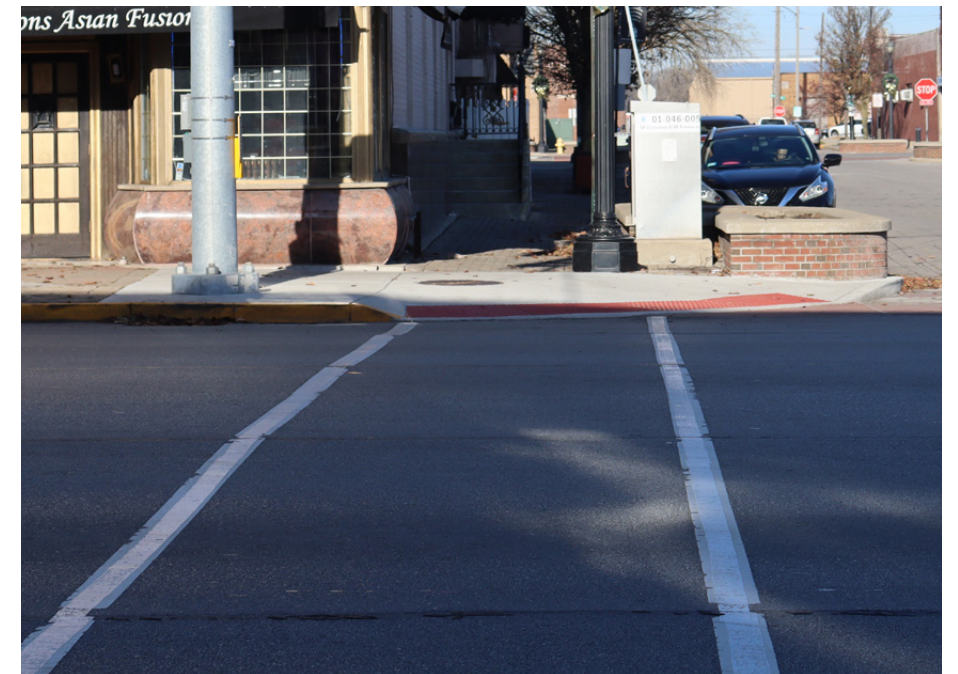
Existing Condition: Painted crosswalks are adequate, but require periodic re-painting Opportunity: Replace painted crosswalks with decorative paving to create consistent pedestrian crossings
