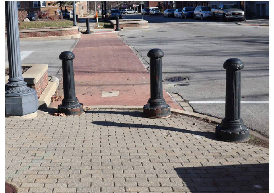
Existing Condition: Bollards used at intersections, singular or in groups Opportunity: Replace with new city standard
