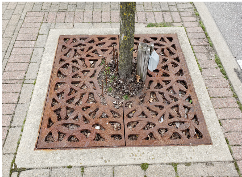
Existing Condition: Trees in tree grates, conditions vary, some missing Opportunity: Replace tree grates with raised planters, new tree grates, or silva cells
